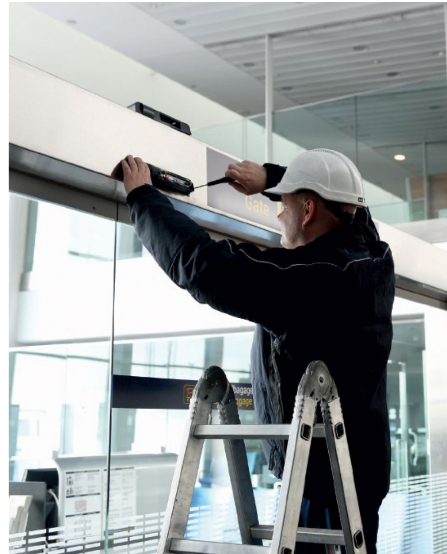
Maintenance in accordance with the manufacturer's specification shall take place at least: "once per year" for all power operated doors and "twice per year" for escape power operated doors.
